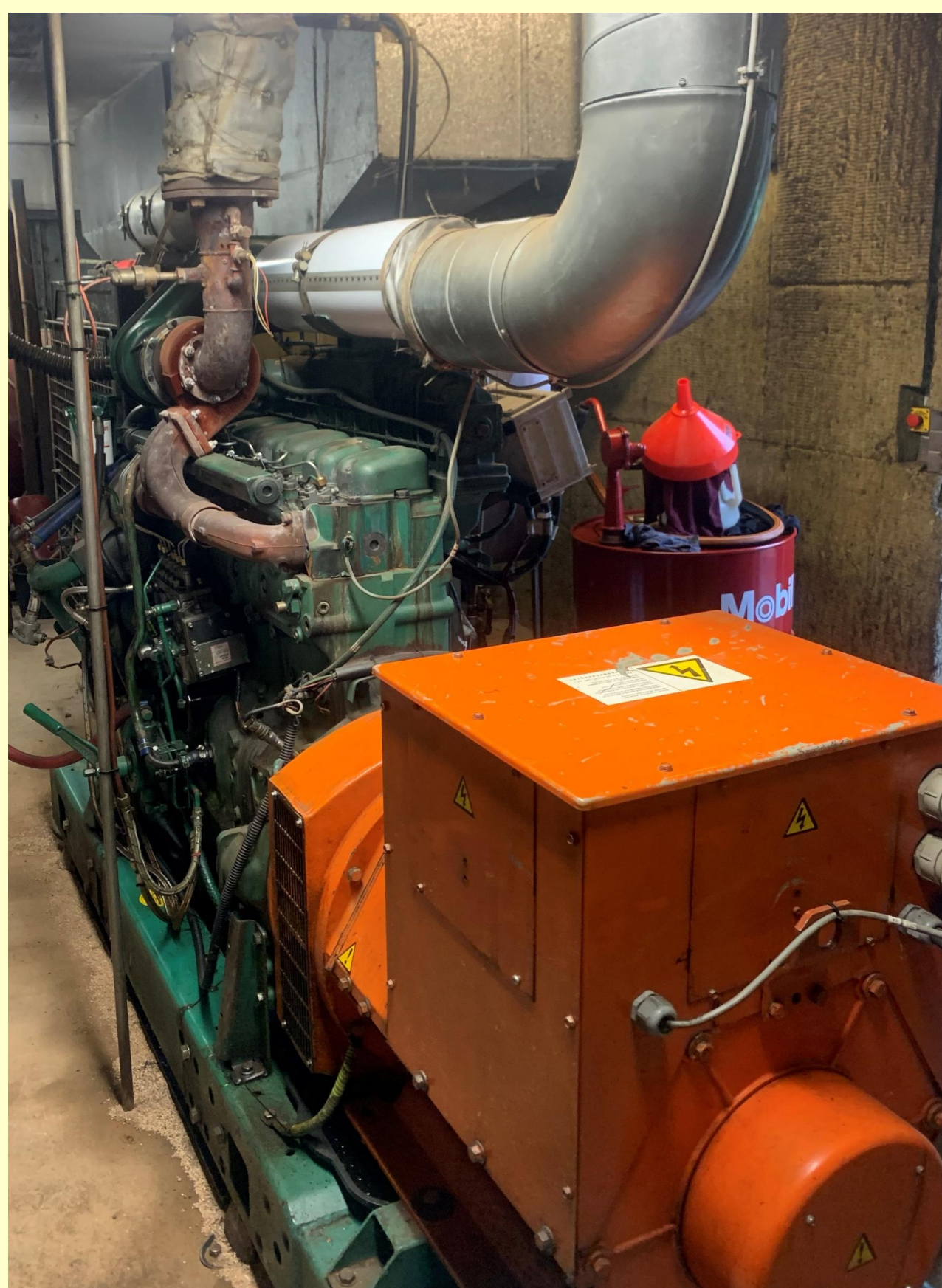
Figure 1. A dual fuel engine at Hedeland, Denmark, using landfill gas as main fuel and diesel as pilot fuel.
